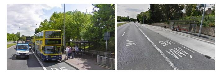
**Figure 1.5** Stillorgan QBC with high bus flows and no bus laybys resulted in bus bunching/ platooning; bus lay-by's provided at key locations to allow express buses to pass slower buses. (Source: Google Maps)
